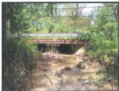
Photograph of Meridian Road Bridge at Damon Run
